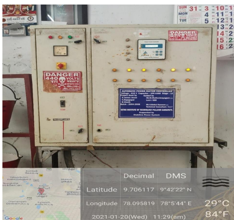
Automatic Power Factor Controller at Power House
